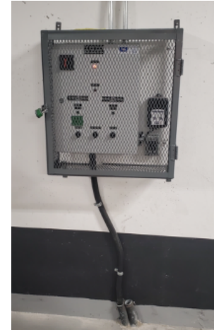
Single OR Double-Door Control Enclosures (with expanded mesh)
