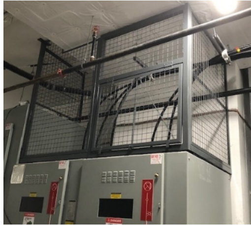
Hydro Approved Hi-Voltage Electrical Enclosures with Access
